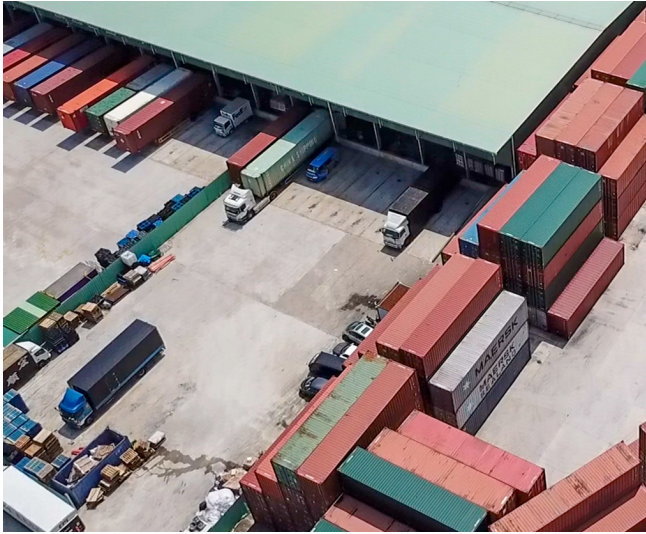
(Figure 38) Warehouse on “Brownfield”
